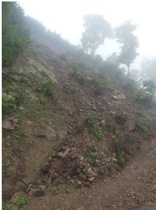
Landslide caused by the road
